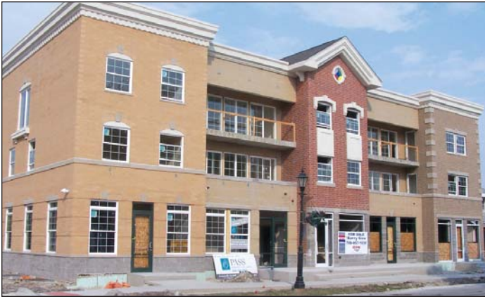
The PASS building, a mixed-use development, is under construction and slated for completion late this summer.
